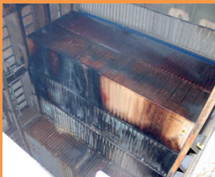
Example of severe fire damage to containers that can be caused by a charcoal fire.
