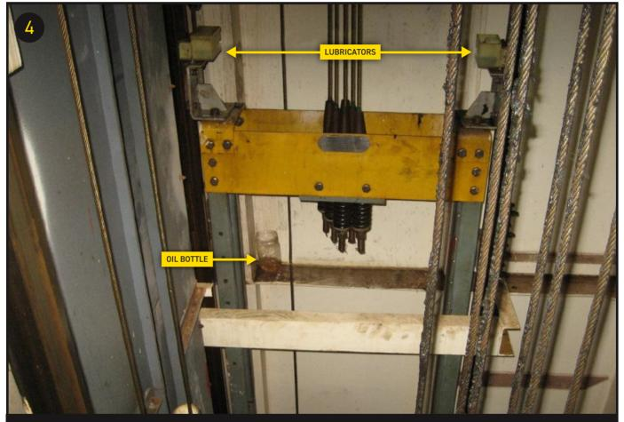
FIGURE 4 POSITION OF LUBRICATORS AND PLASTIC OIL BOTTLE LEFT IN THE ELEVATOR SHAFT SOURCE: INVESTIGATION REPORT 06/2108 BY TRANSPORT MALTA - MARINE SAFETY INVESTIGATION UNIT
