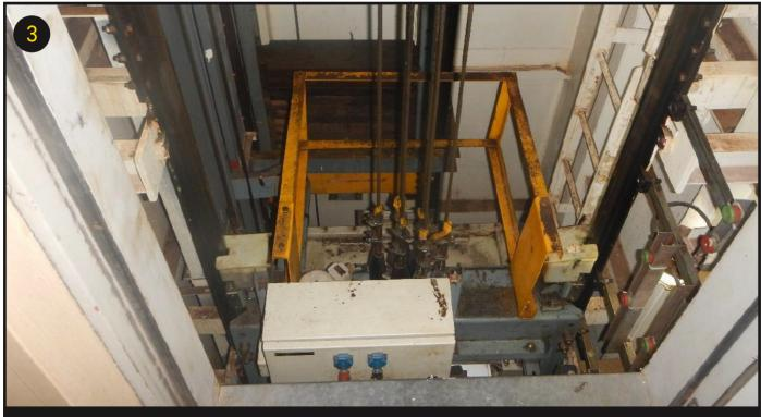
FIGURE 3 TOP OF ELEVATOR CAR SHOWING MAINTENANCE BOX AND SAFETY CAGE SOURCE: INVESTIGATION REPORT 06/2108 BY TRANSPORT MALTA - MARINE SAFETY INVESTIGATION UNIT
