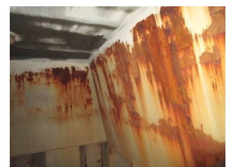
Damaged coating
