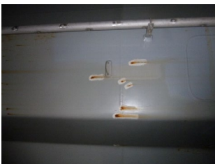
Coating damaged
